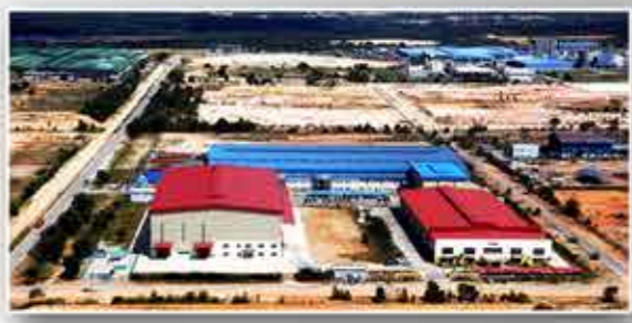
DYNAC SDN BHD main office / factory in Tanjung Langsat, Johor, Malaysia
